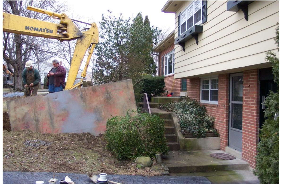
Typical Building Sewer Replacement During Construction
