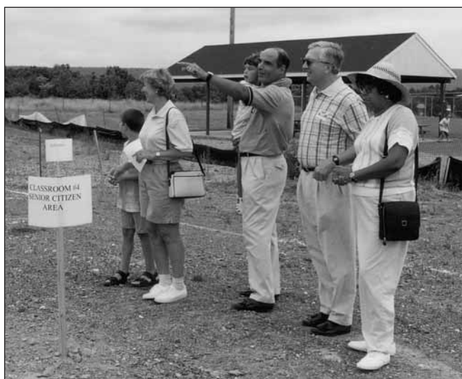
Members of the Community excited to see the building of the Friendship Center underway.
