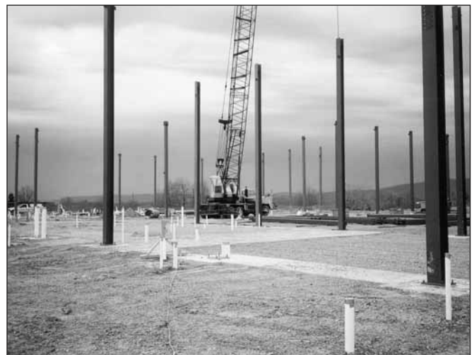
The steel beams — beginning to take shape.
