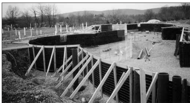
The building of the recreation/therapy pool.
